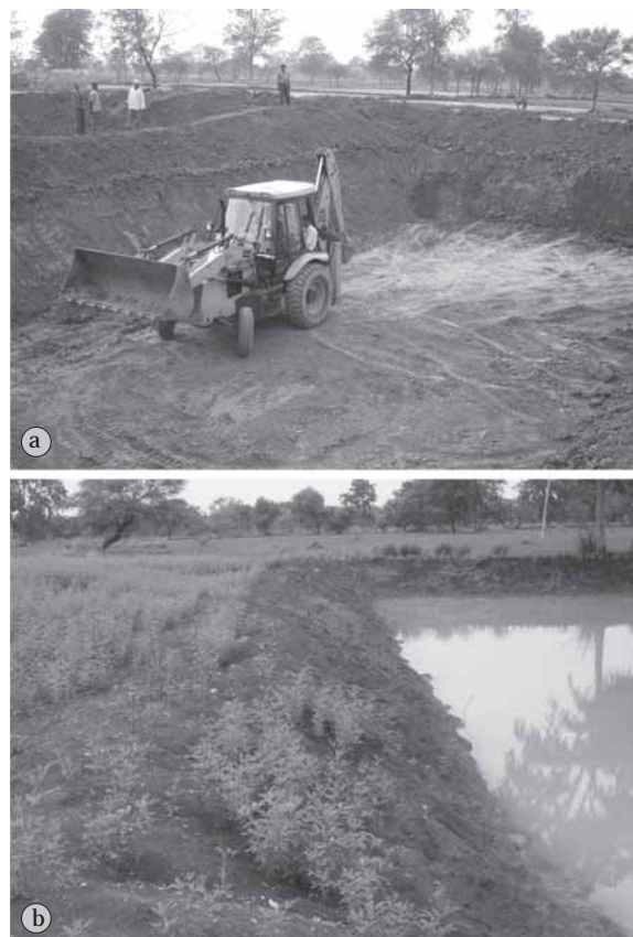
Fig. 1. (a) SFR under construction (b) SFR filled with water and vegetables on the banks
